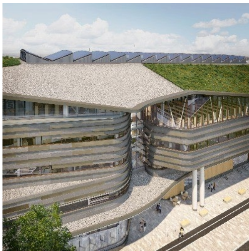
Design drawing of the LAC-OPL joint facility's green roof with solar panels. © 2021 City of Ottawa/Ottawa Public Library/Library and Archives Canada. All rights reserved.
