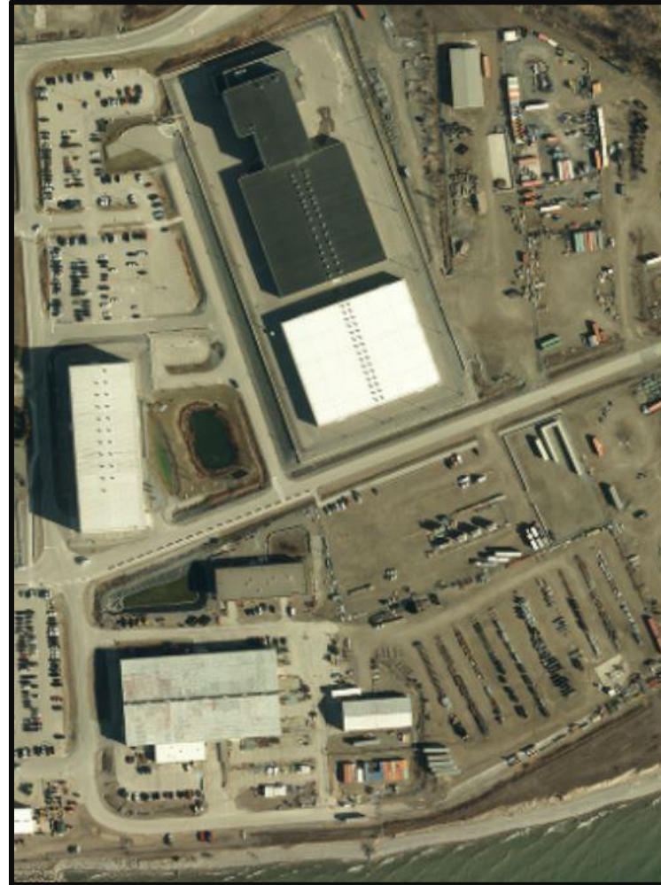
Figure 1.4: Aerial view of the Darlington Waste Management Facility
